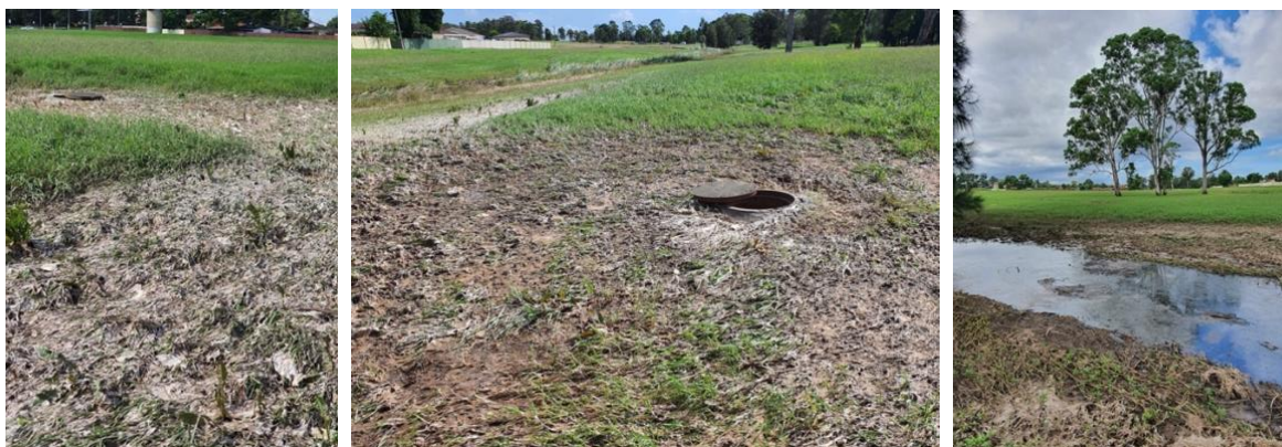
Overflow from the Sydney Water sewer main affected the site in March 2022 (Image: R Howitt)
